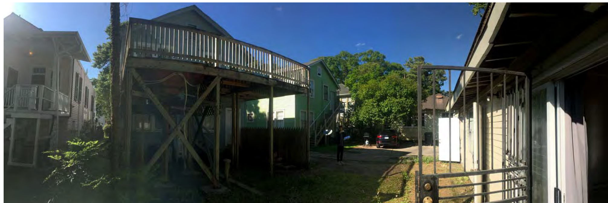
VIEW FROM REAR YARD
